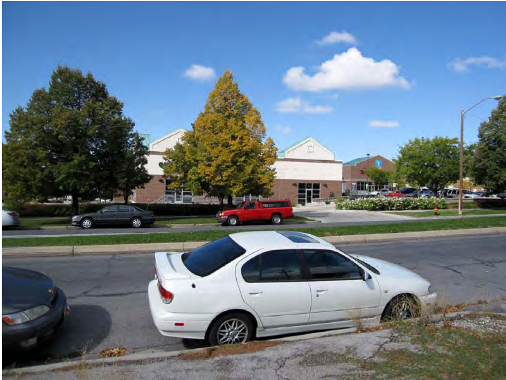
View of building (across 600 East) to the west and located next to Smith's Marketplace.
