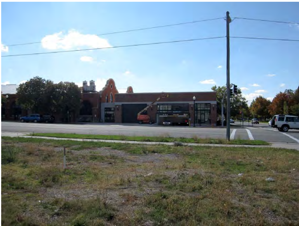
View of Trolley Square (looking south) taken from the subject property.
