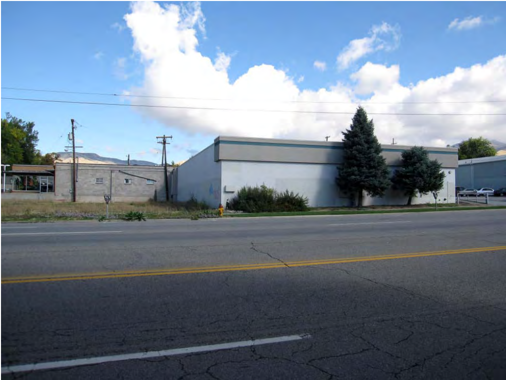
Looking north from across 500 South at building located directly to the east of the subject property.
